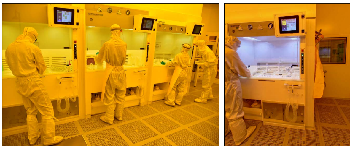
Figure 27: Fume Hoods in the Chemical lab
