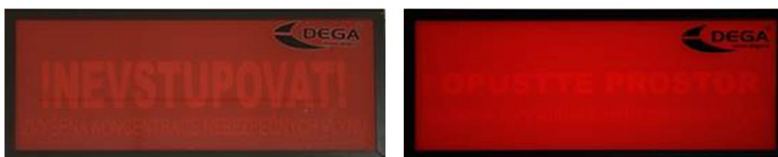
Figure 34: Signal panels are activated when alarm level is reached.
