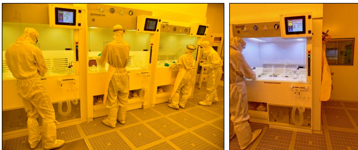
Figure 27: Fume Hoods in the Chemical lab
