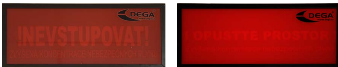
Figure 31: Signal panels are activated when one of the alarm levels is reached:
